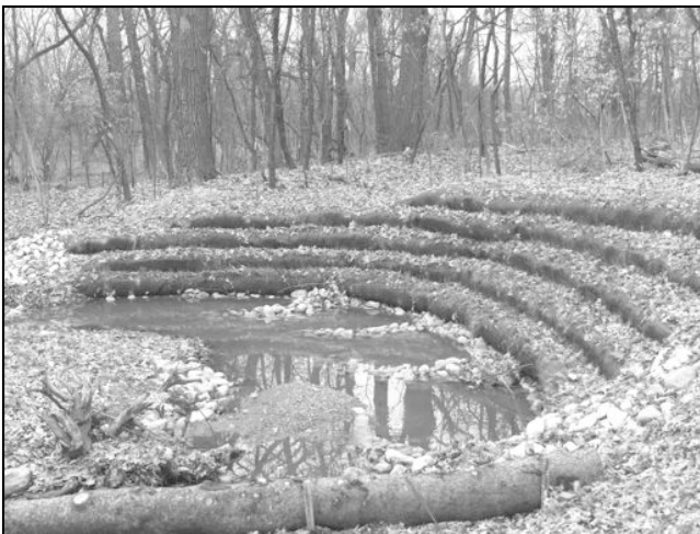
Lyman Woods streambank stabilization, second project site area
