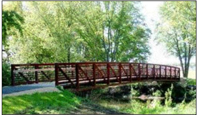
Bike trail truss bridge with an open grated deck
