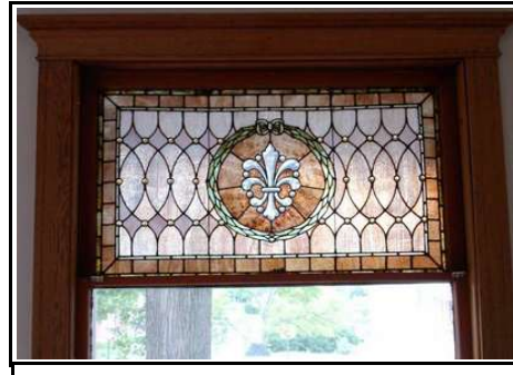
Edwards House window detail
