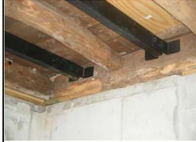
*Hand-hewn joists contrasted with new steel support beams*
